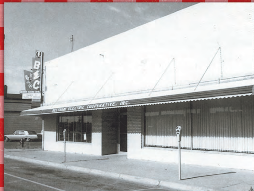
BEC Headquarters at 301 America Ave., Bemidji, MN
