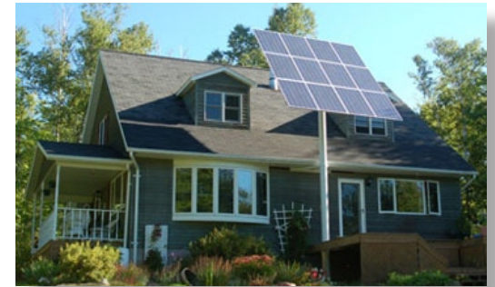
A house in Finland, MN that has a solar electric system in the front yard which generates enough electricity to power most of the home's energy needs. The system is grid-connected and excess energy is sold back to the utility company.
