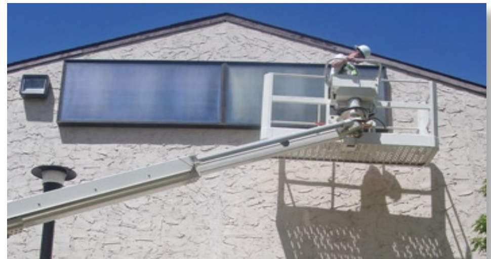
A solar hot air installation at the Little Earth Housing Development in Minneapolis.
